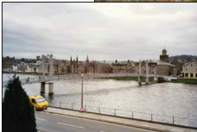
Bridge over River Ness
