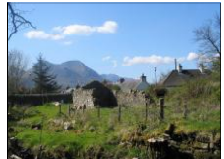
Meal Mill Prior to Repair
